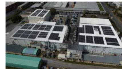
PrimaFineFoods Co., Ltd. Solar power generation facilities
