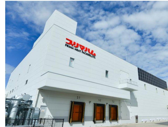
Solar energpower system
