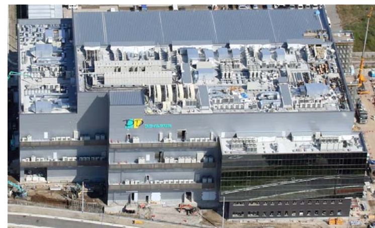
Second Sagamihara Factory under construction
