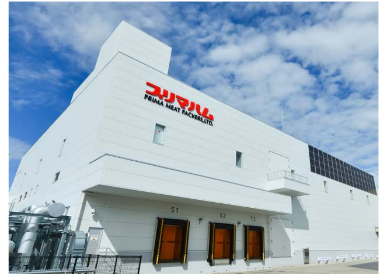
Solar power system
