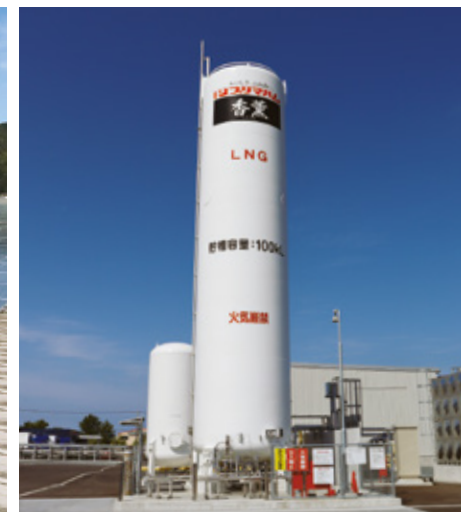
For boiler fuel, the plant uses LNG, which has a low carbon footprint.
