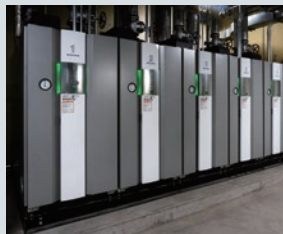
LP gas boiler
