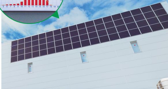
A solar power generation system utilizes wall space, and an information monitor shows how much energy is being generated and saved.
